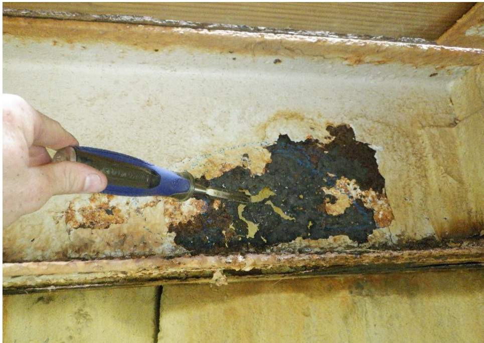
FLOORBEAM 2- 5" HOLE BTW STR 2/3
